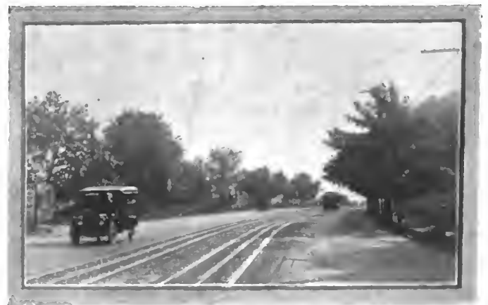
L—The surface of the Yonkers road has been worn smooth by automobile tires
